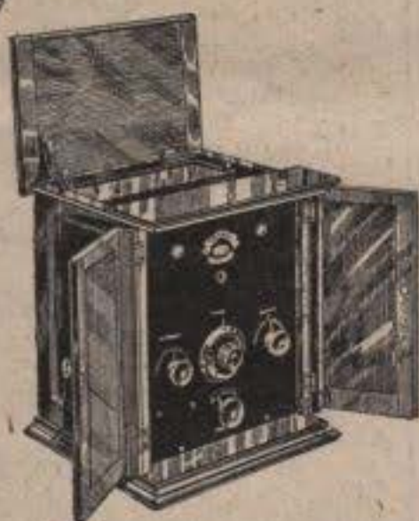
This shows the Sparta Model "A" Receiver with lid opened to give access to high-tension battery and plug-in coils.
